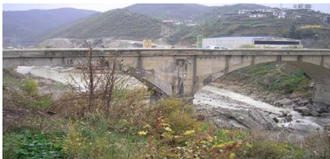
Figure 2: Beshiri Bridge over the Erzeni River – side view
