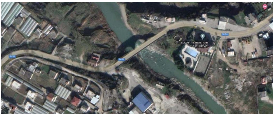
Figure 3: Beshiri Bridge over the Erzeni River – top view
